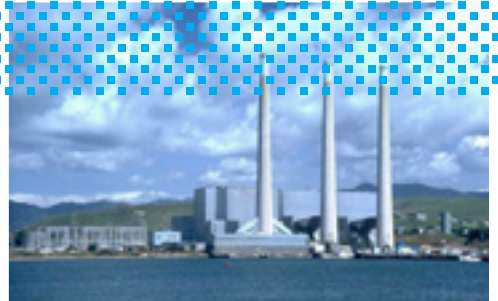
Typical power plant
