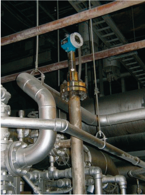
Levelflex M FMP45 installations on feed water heaters
