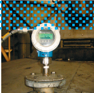
FMP40 mounted on vessel
