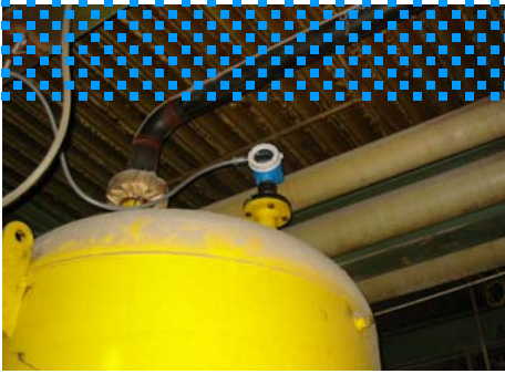
Micropilot M on an acid vessel
