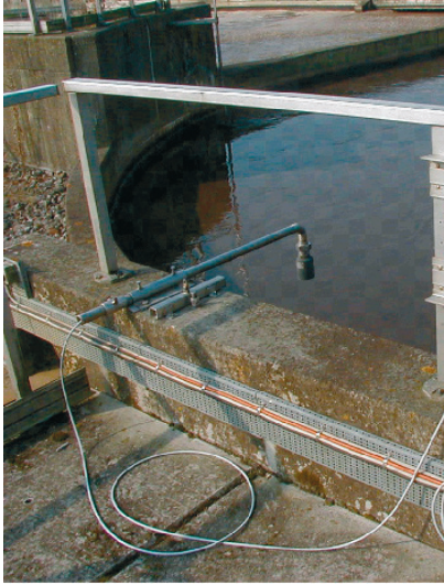
FDU91 sensor mounted over basin
